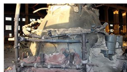
out of pit and cleaning
